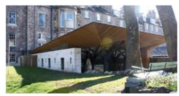
**Frameless glazing - George Square Lane**Glazing is used to create the effect of a floating roof on this building.
