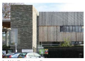
**Careful detailing—Arboretum Place**The timber cladding overhangs cladding on lower levels of the building. This helps shed water from its surface, and protects it from adverse weathering.
